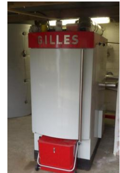
Fig 1. Heating Controls Fig 2. Biomass Boiler
